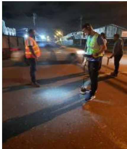
Pinpointing valve location
